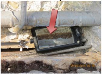
Existing steel which needed to be cleaned and coated was not properly cleaned (wire-wheeled) and coated on the underside...
